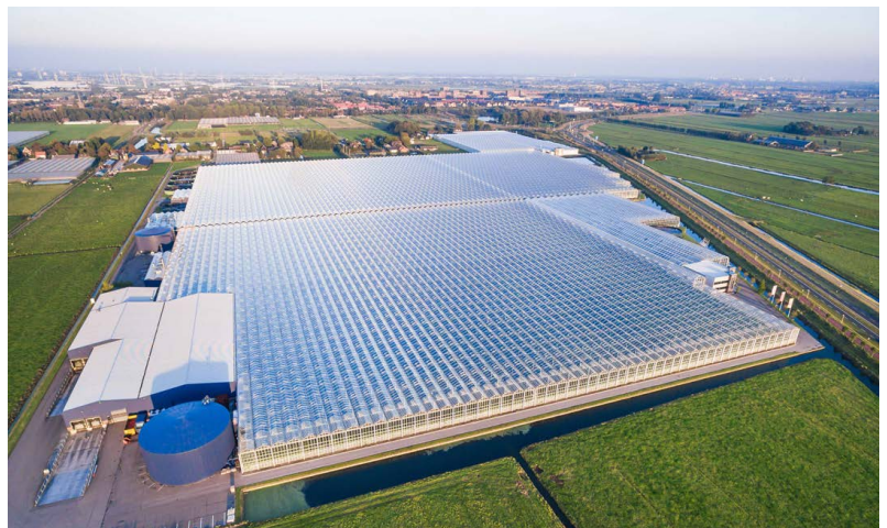
Tomato grower Ted Duijvestijn, main photo, has received finance from Rabobank to invest in geothermally heated greenhouses (right).
